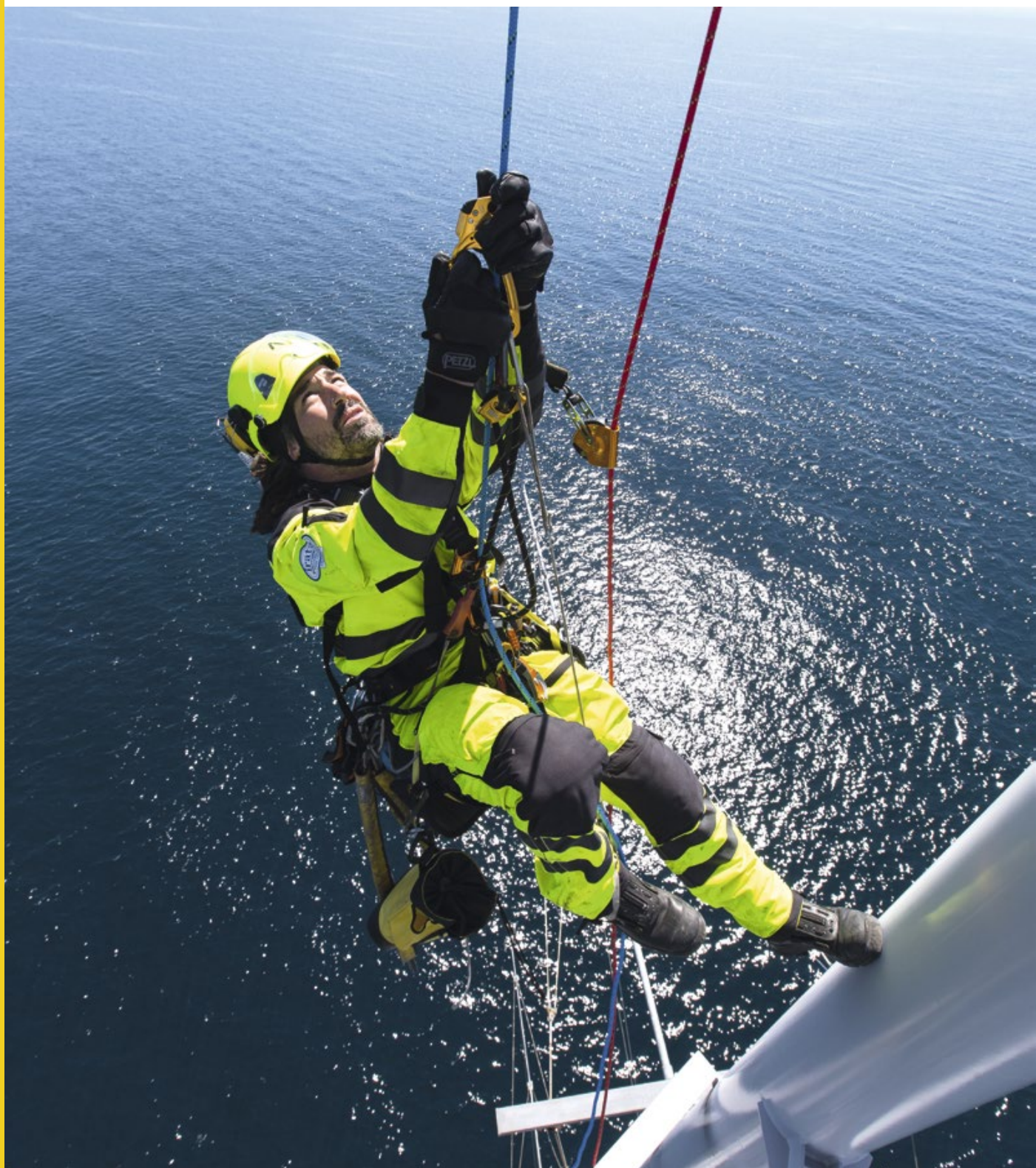
Maintenance Moray Met Mast, Wick, Scotland. © Petzl / vuedici.org / Asaken Rope Access
