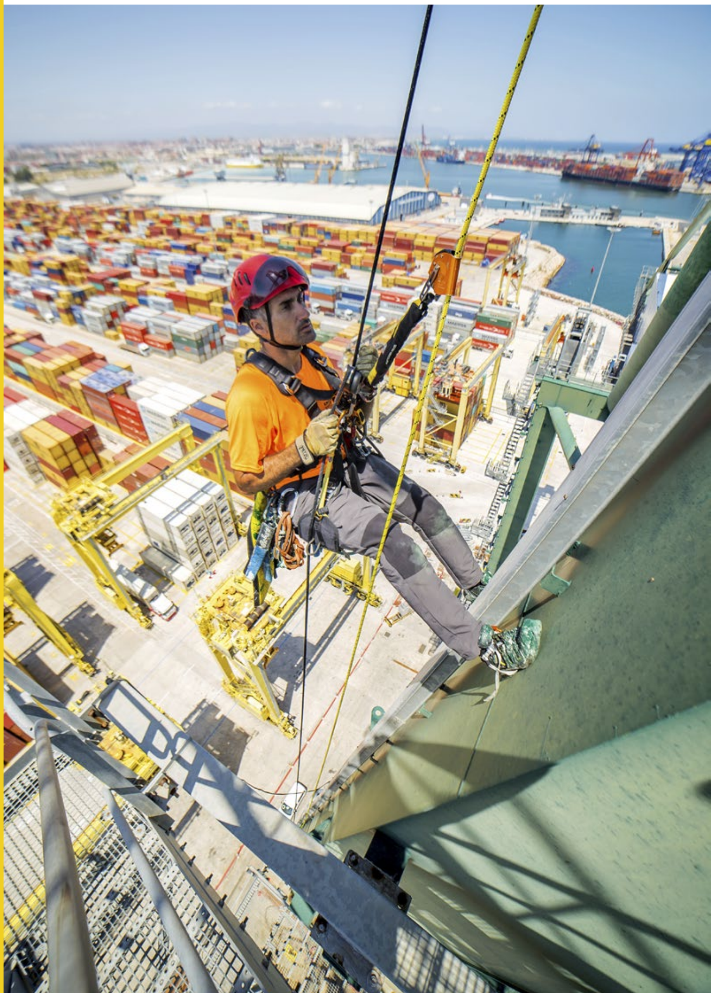
Paint job for the cranes of the merchant harbor of Valencia, Spain. © Petzl / Jan Novak photography / Verice Vertical™
