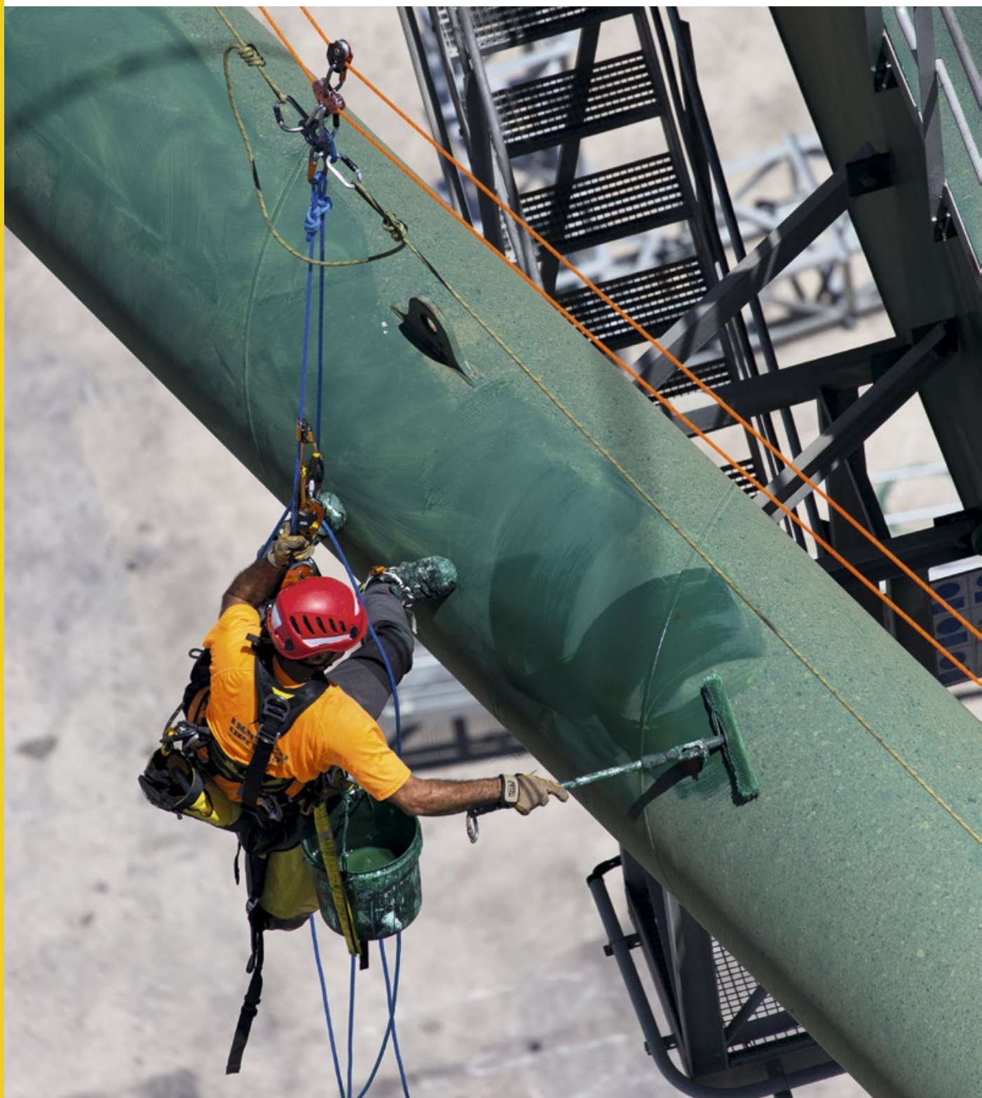
Paint job for the cranes in the merchant harbor of Valencia, Spain. © Petzl / vuedici.org / Vertice Vertical™
